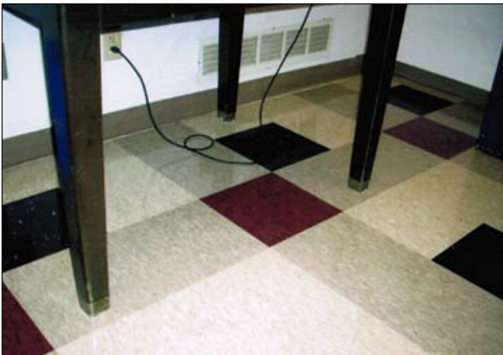
The curtain grouting contractor guaranteed he would stop the water in the classroom building. He did, in only four days, and in time for the new school term.
