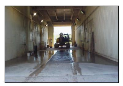
Washwater in the 100-ft. long wash bay flows down through a grate into a pit that gravity feeds to a grease-trap sump. The water is pumped from there into the EC System.
