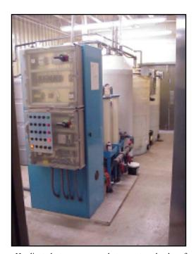
pH-adjusted stream moves between two banks of electrocoagulation cells, where it is exposed to a controlled electrical current. Charged contaminant particles bond together. Masses comprised of emulsified petroleum elements float, while masses containing heavy metals settle.
