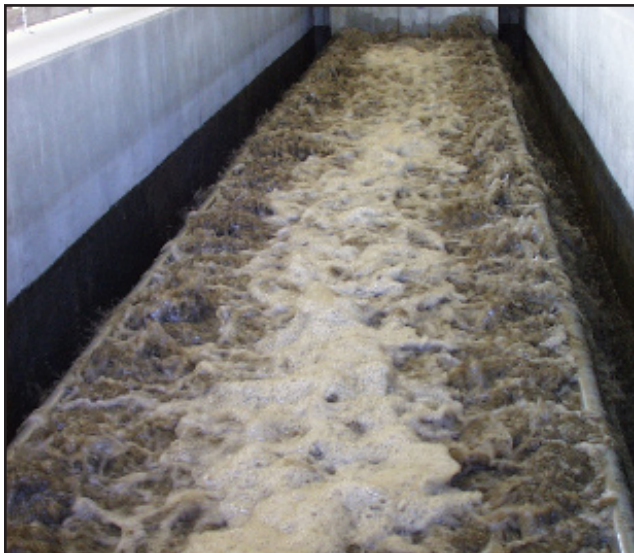
Combined air/water, sustained, sub-fluidized backwash cleans the media, with backwash water consumption as low as 2% of the forward flow.
