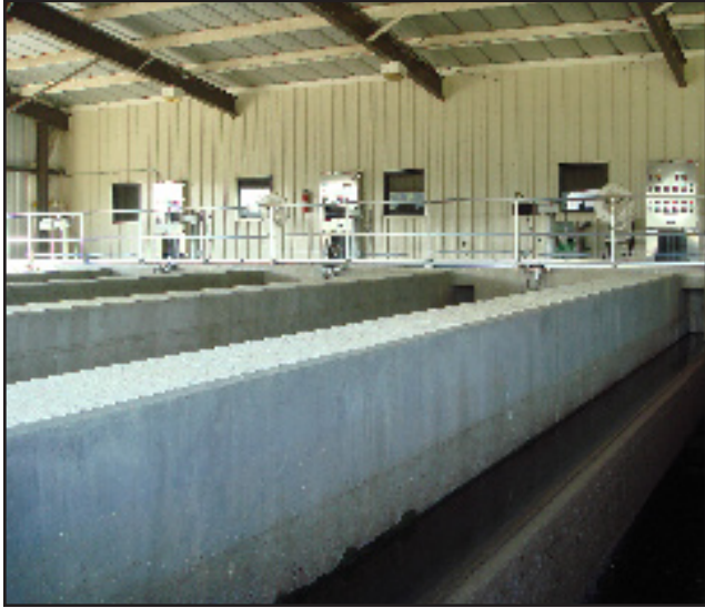
Special, deep-bed biofiltration system is credited with key contribution to utility's continued compliance with state total nitrogen limits, despite ongoing rapid growth in service demand.
