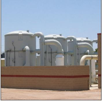
The system consists of nine cells, each containing three trays of media, set up as three towers of three cells each. Design flow per cell is 1000 cfm. The three towers were installed over the 48" influent pipe on the south side of the headworks building.
