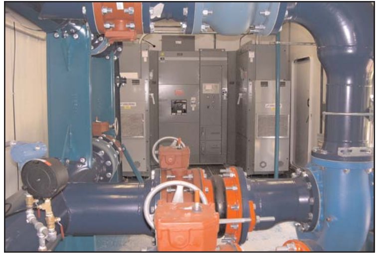
Each skid-mounted, fully integrated pump station included factory-assembled and tested controls.
