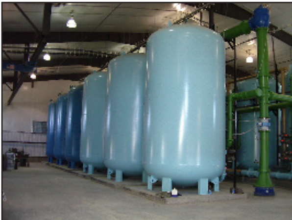
The cation and anion vessels operate in married pairs on line according to demand.
