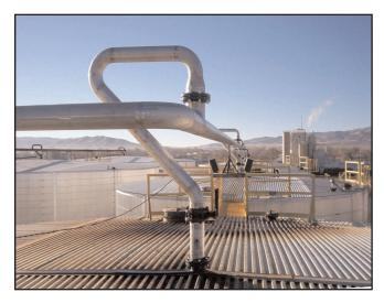
Instead of venting storage tanks to atmosphere, all vapor is collected via pipe from the top of each tank. Original vapors are also collected where trucks are loaded, and where polymer modified asphalt (PMA) is made.
