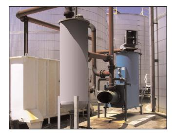
Vapor from the top of each tank is run through a common line to a scrubber. The dewatered vapor then moves to a smoke-removing filtration tank, and then finally to a pelletized AC unit, where all odor is adsorbed.
