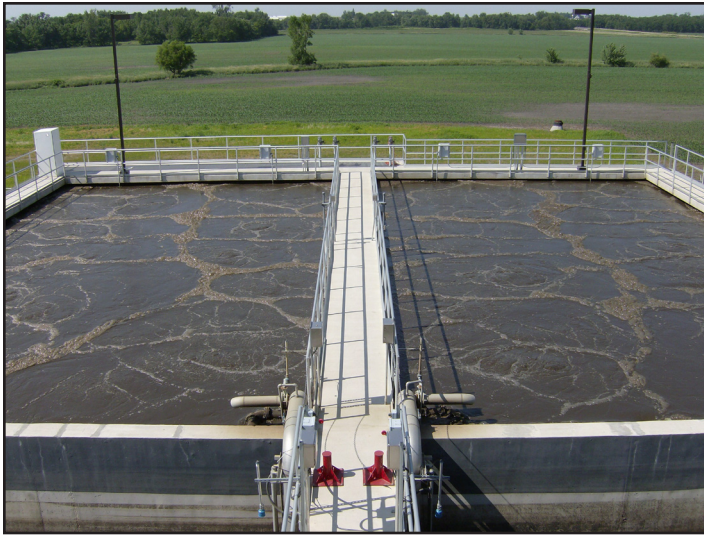
SBRs have rapid fill to operate at maximum water level during interact, in order to increase oxygen transfer and reduce power.
