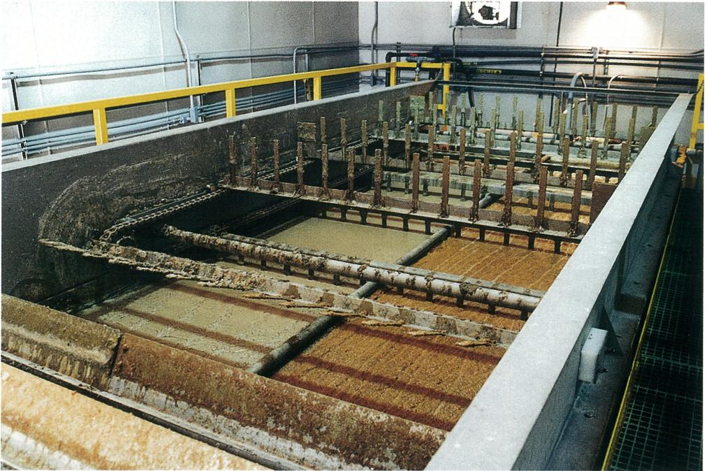
**Second stage of DAF pretreatment:** unique horizontal, open-style “split” DAF cell receives water on one side of the unit for treatment, and discharges effluent to an activated sludge tank. Discharge from the activated sludge tank feeds back to the other side of the “split” unit for further treatment before being gravity fed to the city sewer.
