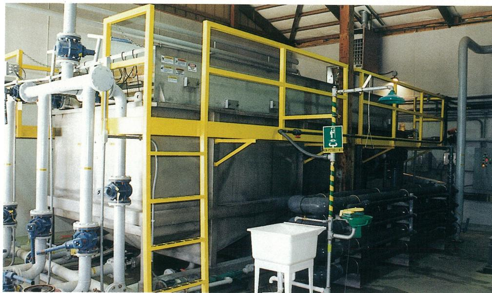
Marburger Foods Inc.’s Peru, IN pre-cooked bacon processing operation salvages fat for sale at an average rate of 35,000 lbs/wk., through use of dissolved air flotation (DAF) wastewater processing units. The units also assured continued municipal discharge compliance for projected wastewater flow increase from plant expansion.
