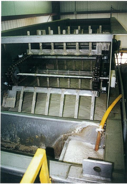
**First stage of DAF pretreatment:** twin vertical, lamella plate-style cells treat 35,000 gal./day of wastewater each. Fat is skimmed off and pumped to a tanker, with the effluent pumped to a common flow equalization tank before being pumped to second-stage treatment cell.
